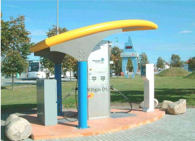
**Fig 3. Dispenser hydrogen and mix of CNG/hydrogen**
