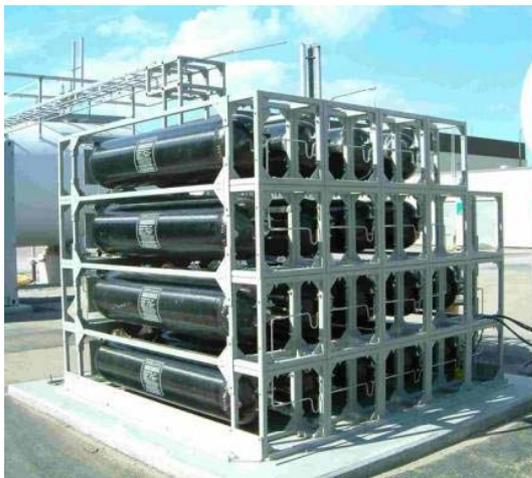
Fig 1. Hydrogen storage pressure tanks
